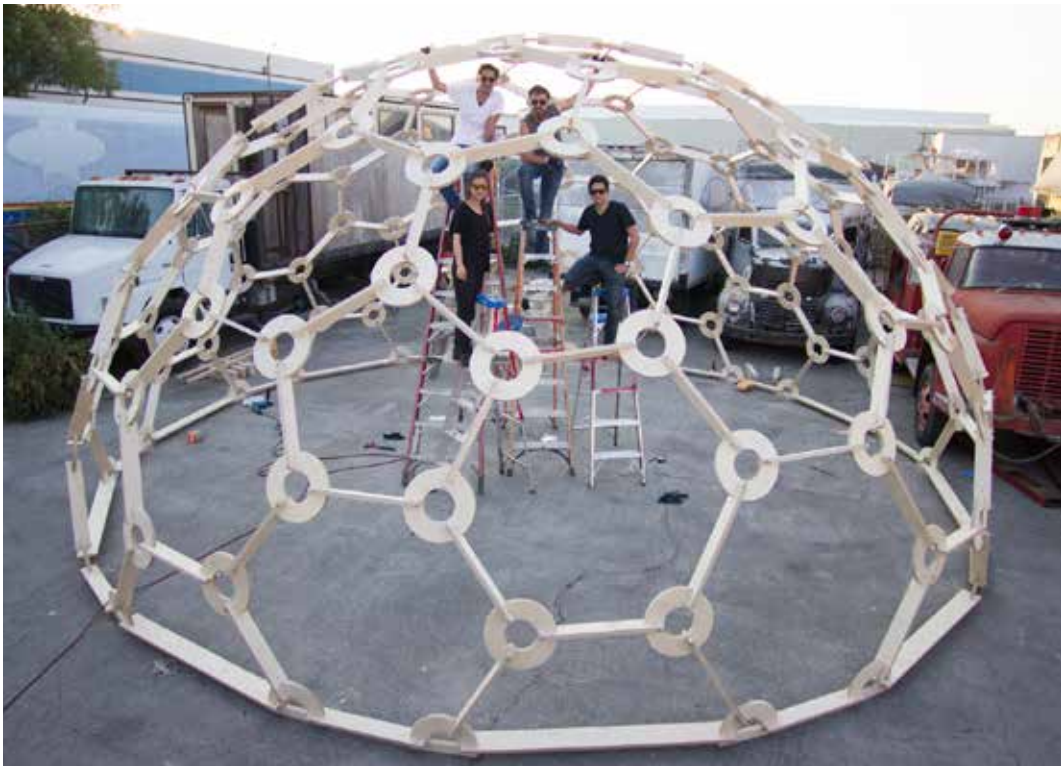
FIG. 2.31 Prebuilding the construction of the dome "desert eyes", 2017. (image: J. Booth)
