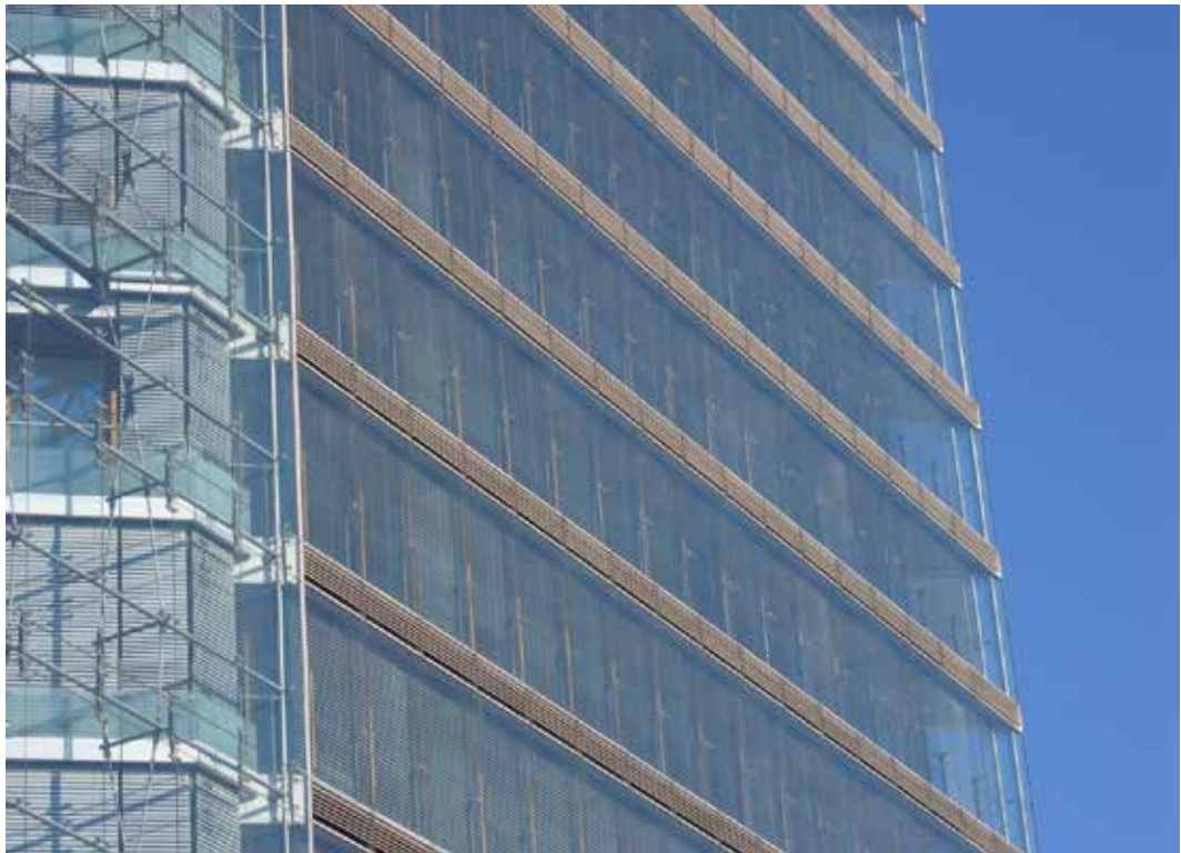
FIG. 3.5 Stadttor Düsseldorf with one of the early double facades (image: U. Knaack)
