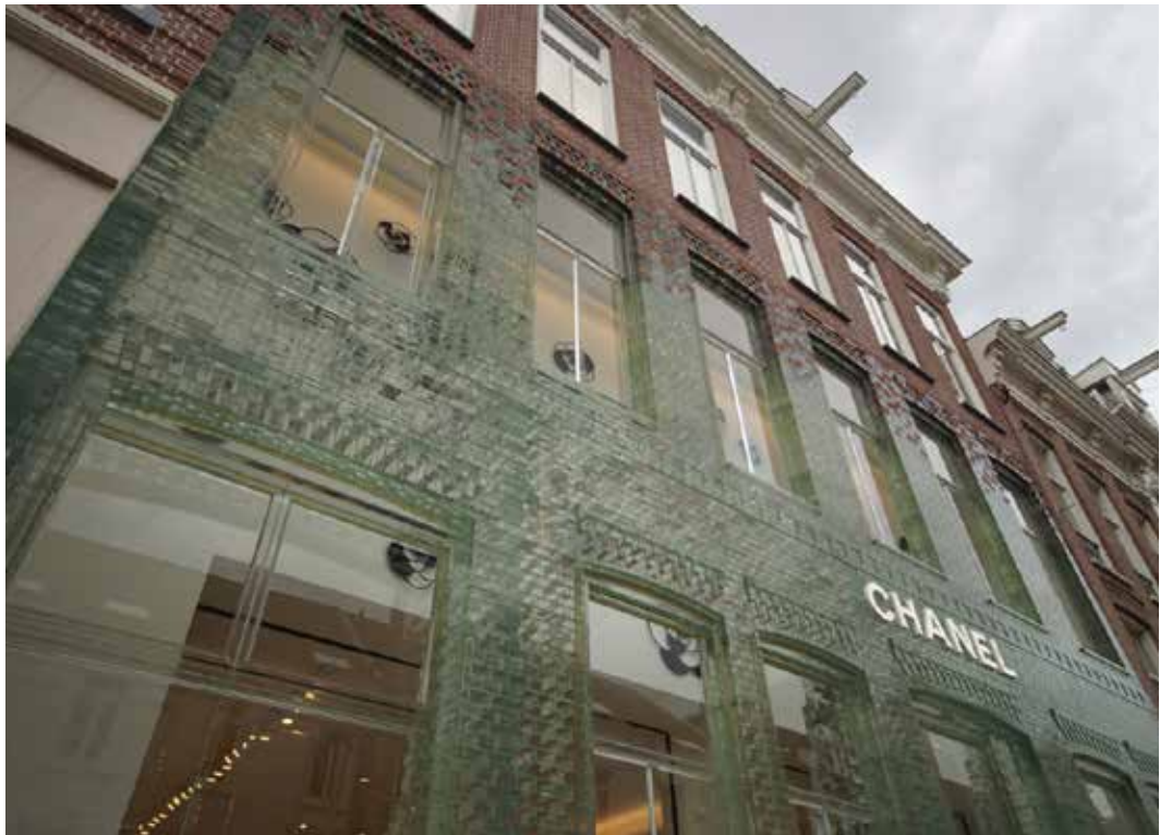
FIG. 3.9 Glass Brick Wall of the PC Hooftstraat shop in Amsterdam, developed by the TU Delft Glass Team around Prof. Rob Nijse. (image: U. Knaack)
