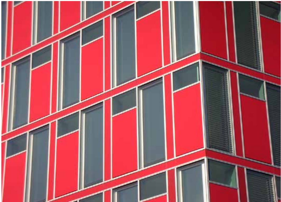
FIG. 3.7 Capricon Building Düsseldorf – one of the few build component facades (red areas). (image: U. Knaack)
