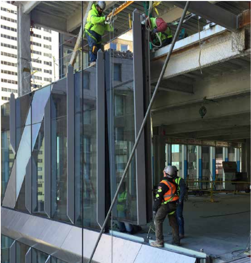
FIG. 2.11 The Comcast Building in Philadelphia (2016) shows a high degree of prefabrication with unitized facade elements that allow for a faster assembly but also need an efficient logistic and in time delivery. (image: U. Pottgiesser)
