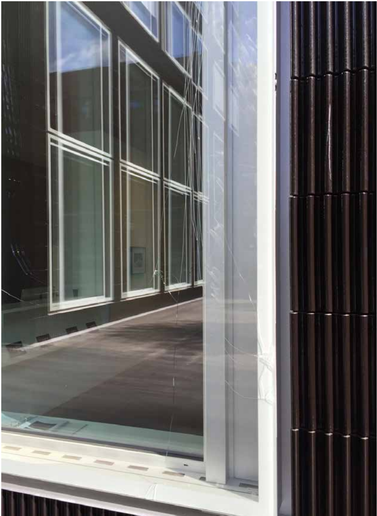
FIG. 2.1 The facades and the details of the Löwenbräuareal in Zürich, Switzerland (by Gigon / Guyer Architects and Atelier WW) show the complexity of present building envelopes in materiality, construction and technology. (image: U. Pottgiesser)
