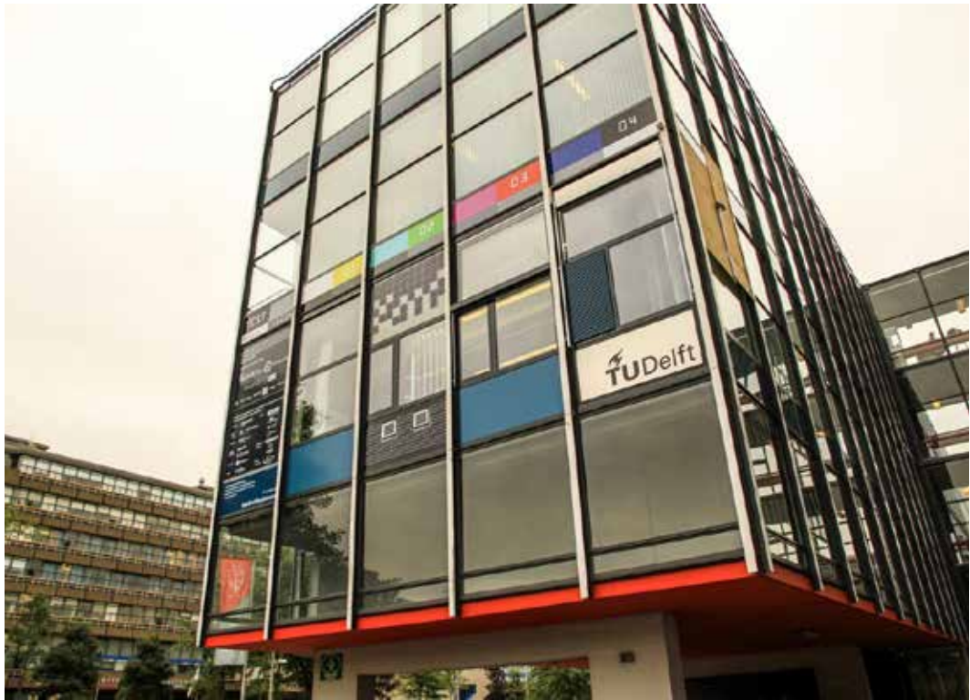
FIG. 3.8 Mockup of the Leasing Façade Concept at TU Delft with 4 different technical solutions to be tested. (image: U. Knaack)
