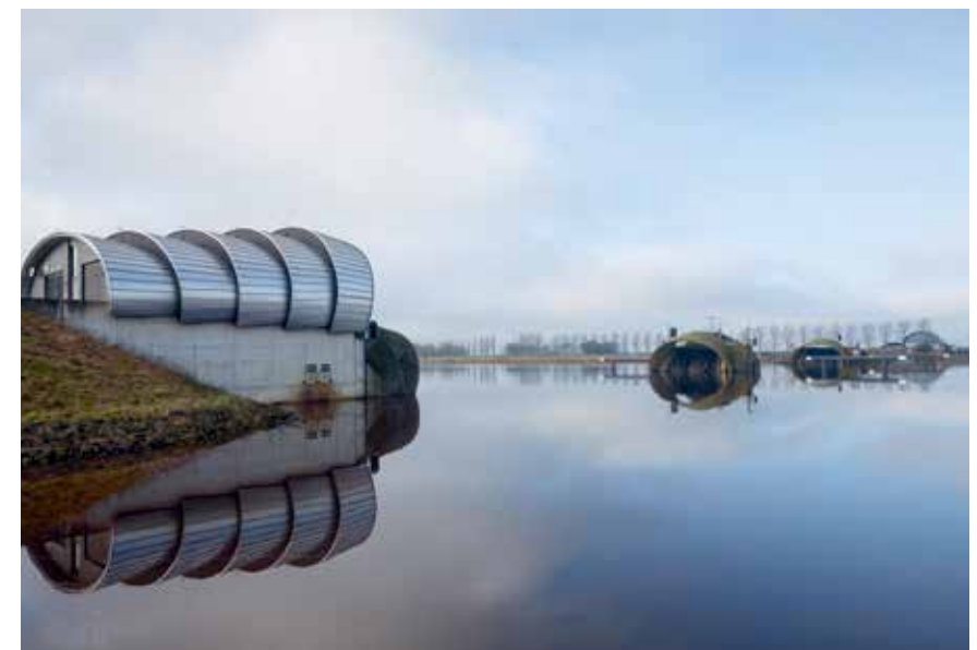
Balgstuw (inflatable barrier) Ramspol, an innovative and flexible way to protect the IJsseldelta against floods.
