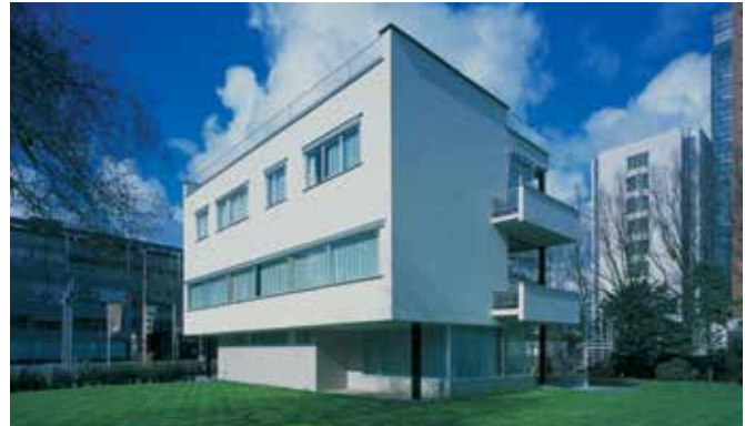
FIG. 2.4 Huis Sonneveld (Brinkman & Van der Vlugt 1933) was also one of the buildings preselected to represent the 1850–1940 period. It was listed in 1986 and is a house museum today / Jannes Linders
