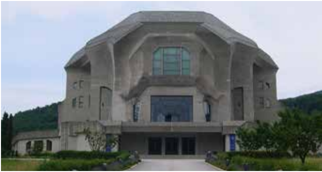
FIG. 3.20 The Second Goetheanum, Dornach. The roof forms an integral part of the sculpture-like design by Rudolf Steiner / Marieke Kuipers
