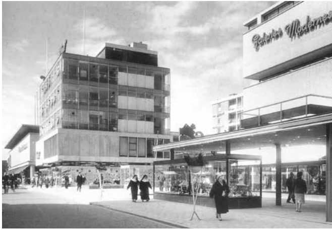
FIG. 5.14 The HUF Building in its original state around 1953 / Gemeente Archief, Rotterdam
