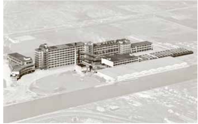
FIG. 5.5 An aerial photograph of the Van Nelle Factory from the 1950s, the original extent of the project highlighted / KLM Aerocarto – Gemeente Archief Rotterdam – overlay by Wessel de Jonge Architects
