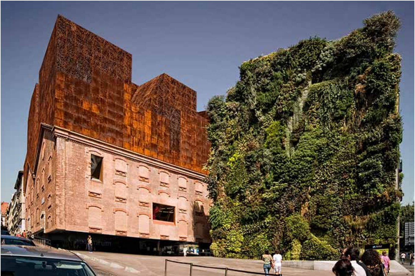
FIG. 2.23 A power station in downtown Madrid after the transformation into the CaixaForum museum by Herzog & De Meuron Architects / Oscar Carnicero. Licensed under Creative Commons. Attribution-ShareAlike 2.0 Generic. Retrieved from https://flic.kr/p/7stYGq
