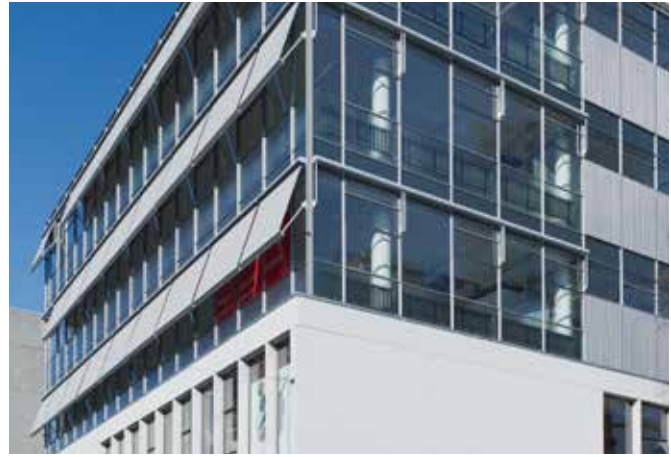
FIG. 5.17 The HUF Building restored in 2009; the newly installed awnings allowed for the use of clear insulated glazing units instead of sun reflective glass panels / Jannes Linders
