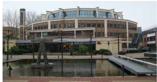
FIG. 3.23 The 16-sided Bouwcentrum, Rotterdam (former exhibition centre on construction), built to the design of Joost Boks, topped by a glazed dome and built with a remarkable reinforced concrete construction expressed in both the interior and the exterior / Marieke Kuipers
