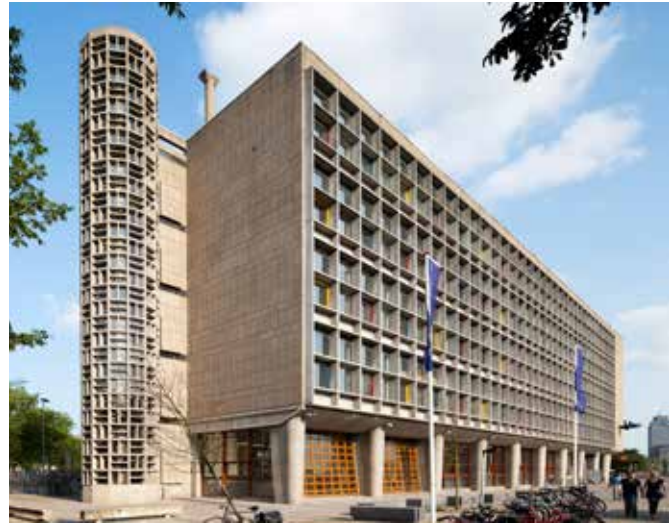
FIG. 5.22 An overview of the Technical School Patrimonium after restoration in 2013, showing the sectional doors of the former car mechanics workshop / Raoul Suermondt
