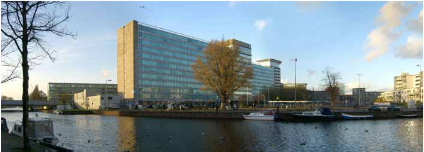
FIG. 2.26 The GAK Building in Amsterdam (Ben Merkelbach, Piet Elling, Alexander Bodon 1960) was abandoned in 2005 / Theo van Leur
