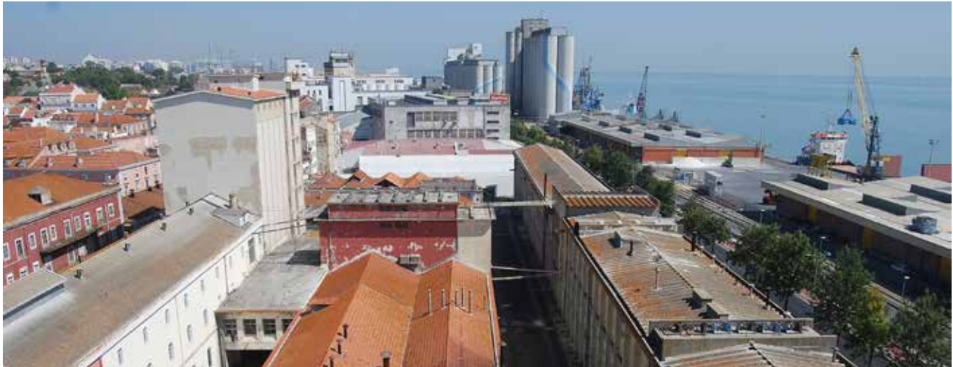
FIG. 4.16 Overview of the Manutencao Militar Complex in the parish of Beato in Lisbon, located parallel to the Tagus River as seen from the top of the complex's silo / Marieke Kuipers
