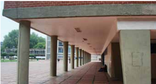
FIG. 3.22 The columns of the concrete skeleton structure exposed on the ground floor level of one of the National University campus buildings (UNAM) of Mexico; the layout of the campus' pavement is also part of a structured design / Marieke Kuipers
