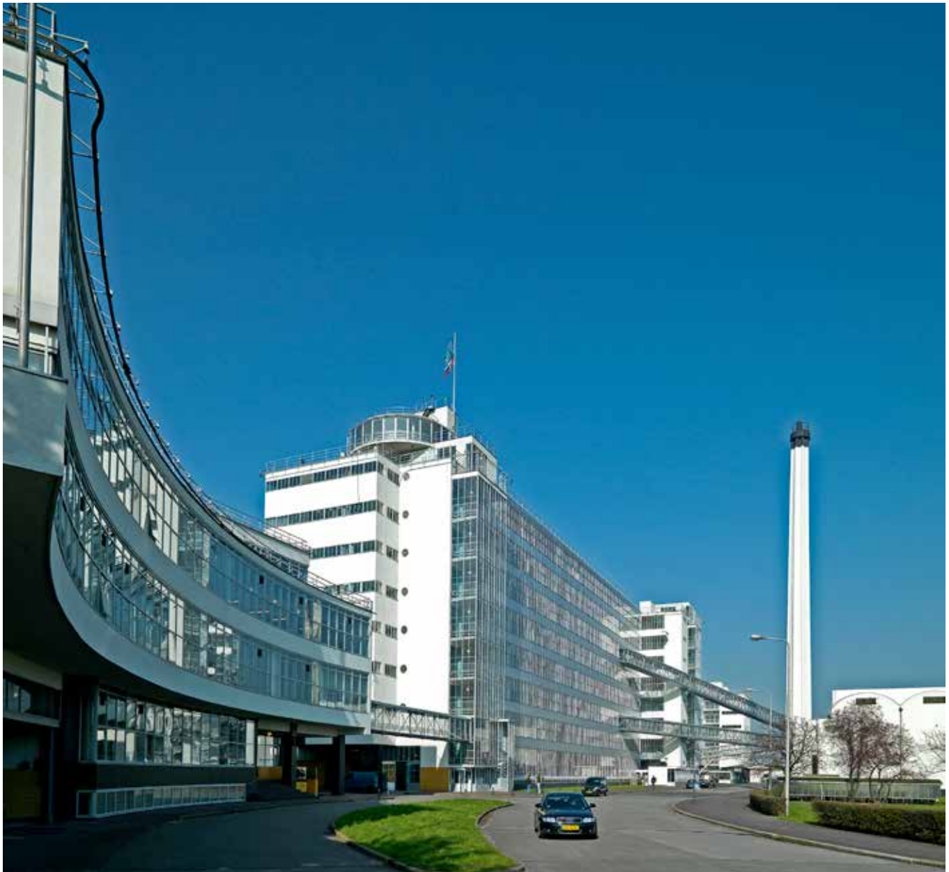
FIG. 5.37 The Van Nelle Factory, documented for the UNESCO World Heritage nomination in 2013 / Fas Keuzenkamp
