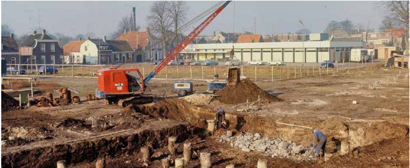
FIG. 3.24 A construction site with old concrete piles exposed, Oosterhout / courtesy of the Cultural Heritage Agency of the Netherlands
