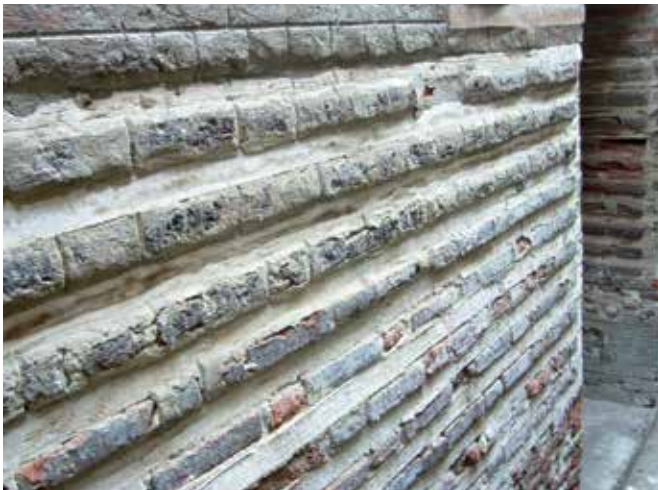
FIG. 3.7 Combination of brick and timber layers in the lower part of masonry walls (building, Coptic quarter, Cairo, Egypt) / photo: R. v. Hees
