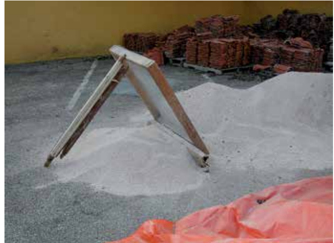
FIG. 4.10 Sieving, even with simple means, results in rather coarse grained sand, as a basis for plasters that turned out to be better salt resistant. The remaining fine sand fraction can be used for other types of plaster and as a filler in other applications / photo: R. v. Hees
