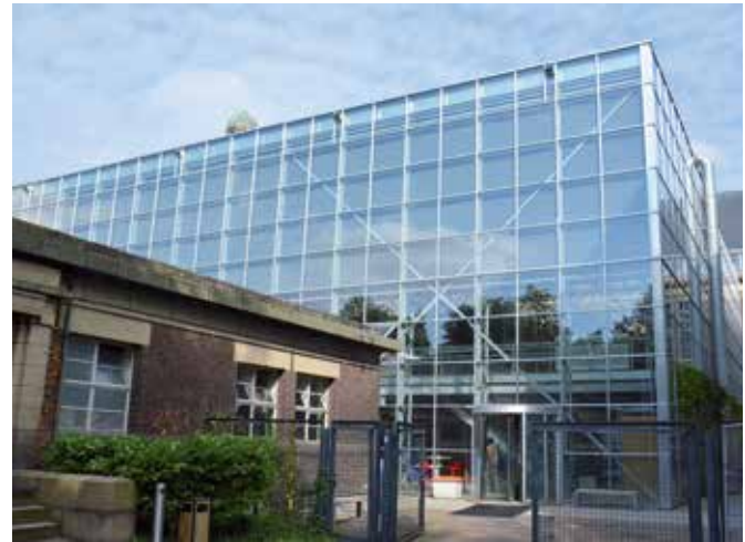
FIG. 6.22 Courtyard transformed into an interior space, exterior (Faculty of Architecture, TU Delft, The Netherlands) / photo: S. Naldini
