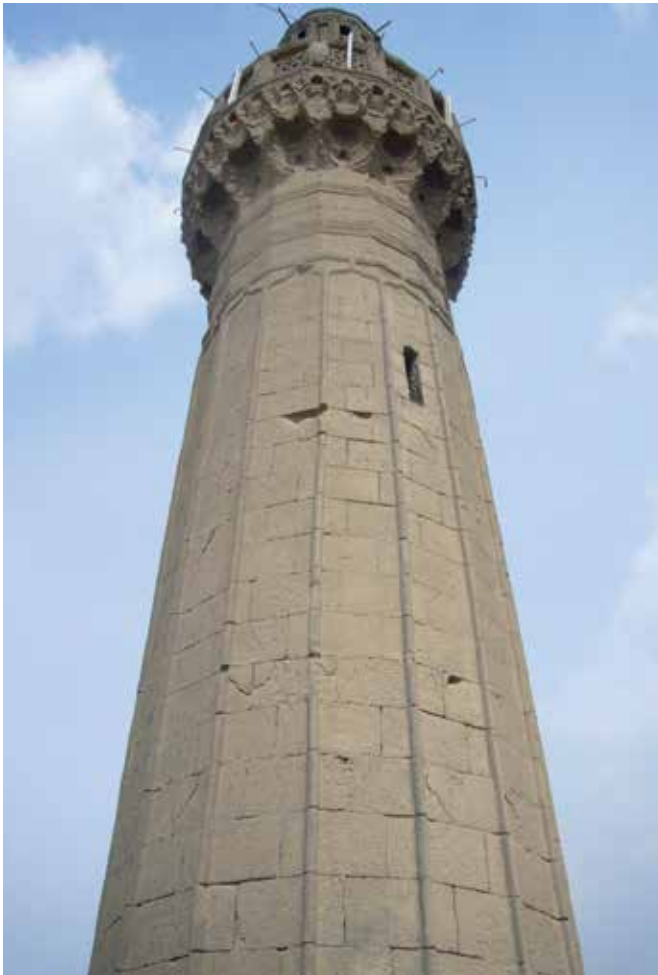
FIG. 3.5 Diagonal cracks in different directions, visible after the 1992 earthquake (minaret, Al Faqahani mosque, Cairo, Egypt) / photo: R. v. Hees
