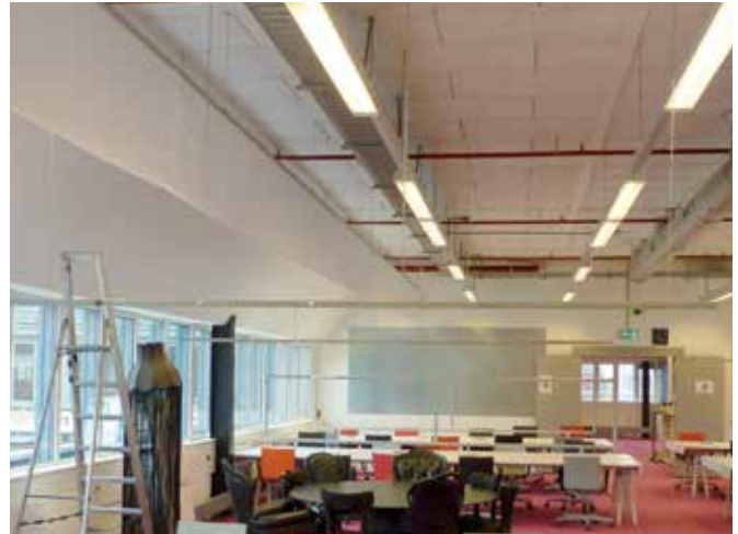
FIG. 6.28 Supply (fabric) and exhaust ducts (Faculty of Architecture, TU Delft, The Netherlands) / photo: S. Jansen
