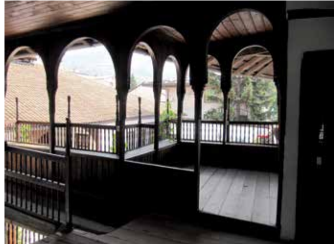
FIG. 5.4 A beautiful and articulated veranda (Svrzo's House, Sarajevo, Bosnia) / photo: S. Op den Kamp
