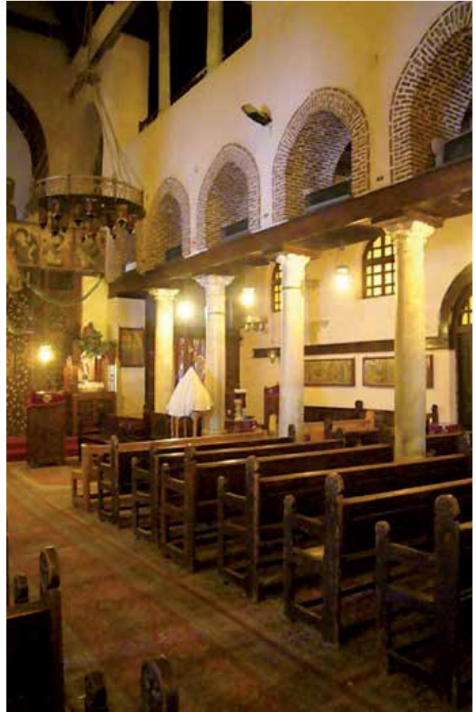
FIG. 3.8 Timber beam supporting the arches and contributing to the ductility of the structure (Coptic church, Cairo, Egypt) / photo: R. v. Hees
