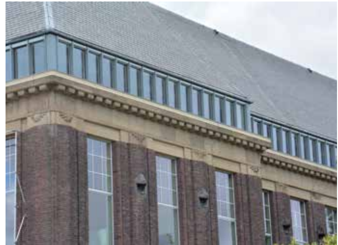
FIG. 6.31 Present situation of roof and windows; the frames are now aluminum (Faculty of Architecture, TU Delft, The Netherlands) / photo: S.Naldini
