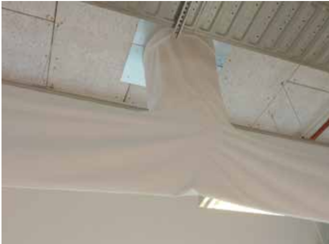
FIG. 6.28 Supply (fabric) and exhaust ducts (Faculty of Architecture, TU Delft, The Netherlands) / photo: S. Jansen
