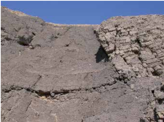
FIG. 2.3 Mastaba, Meidum, adobe (Egypt), detail / photo: D. Schulz
