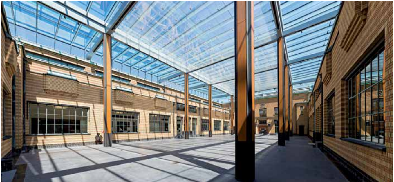
FIG. 6.38 The glass structure floating on the existing walls in the transformed garden (Gemeentemuseum, The Hague, The Netherlands, arch. Braaksmā & Roos) / photo: A. Veldt
