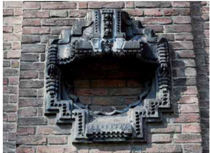
FIG. 6.26 The lion head like ventilation openings (filling visible inside) (Faculty of Architecture, TU Delft, The Netherlands) / photo: S. Naldini
