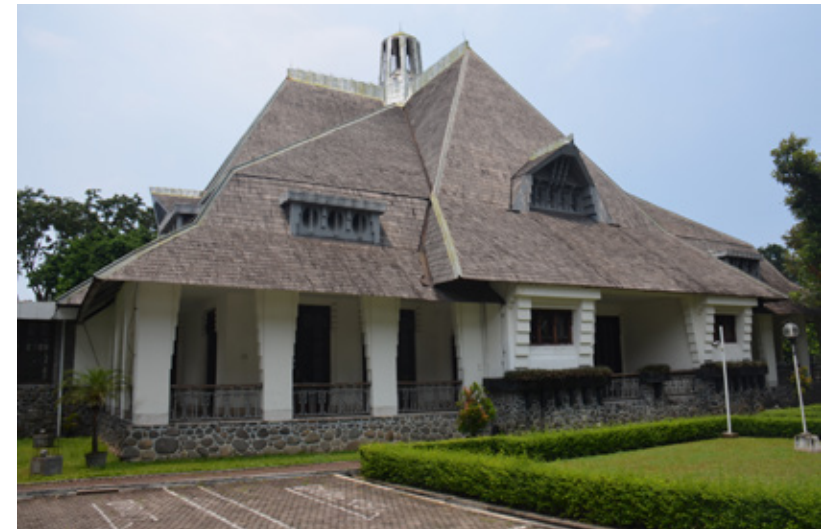
8 — Job & Spreij architectural practice, house for an agent of the Javasche Bank in Surabaya, 1921. Photo by Obbe Norbruis.
