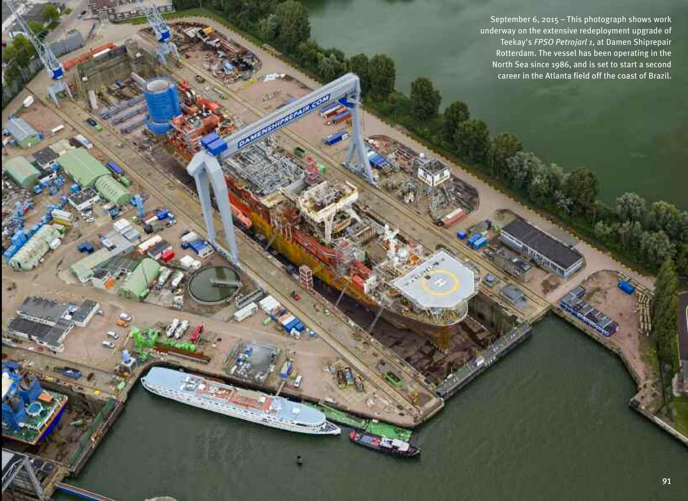
September 6, 2015 – This photograph shows work underway on the extensive redeployment upgrade of Teekay's FPSO Petrojarl 1, at Damen Shiprepair Rotterdam. The vessel has been operating in the North Sea since 1986, and is set to start a second career in the Atlanta field off the coast of Brazil.
