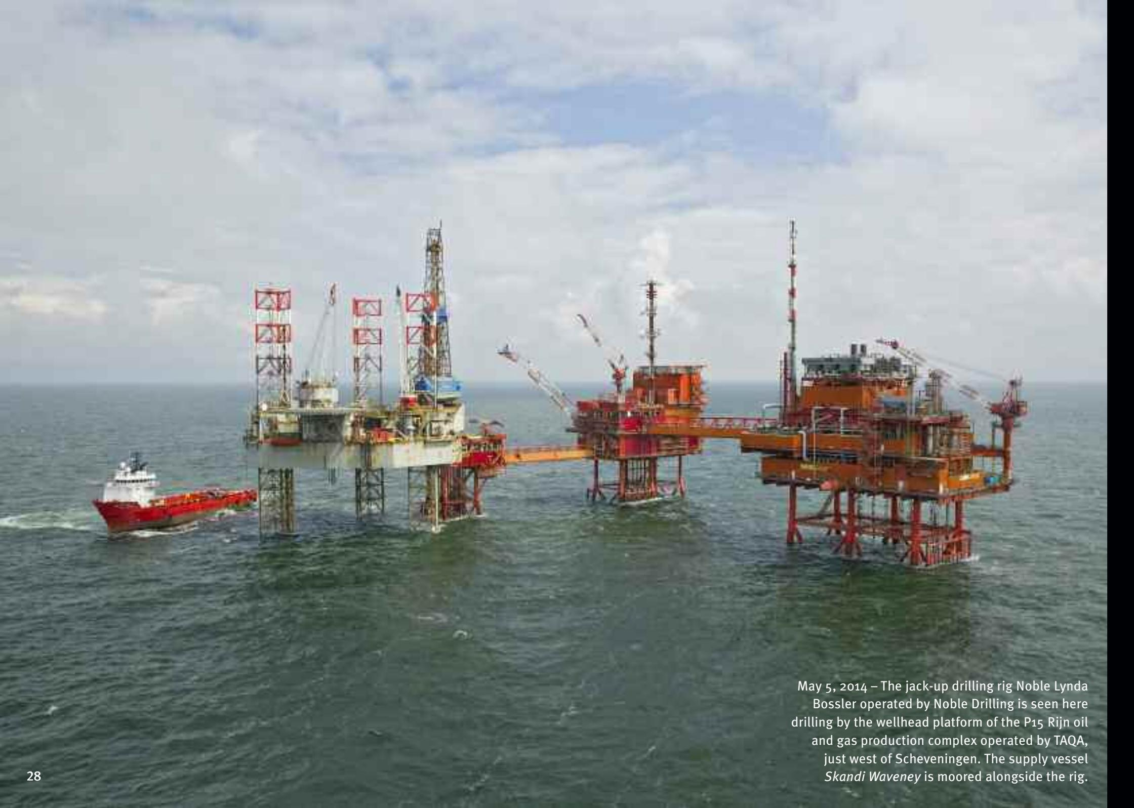
May 5, 2014 – The jack-up drilling rig Noble Lynda Bossler operated by Noble Drilling is seen here drilling by the wellhead platform of the P15 Rijn oil and gas production complex operated by TAQA, just west of Scheveningen. The supply vessel *Skandi Waveney* is moored alongside the rig.
