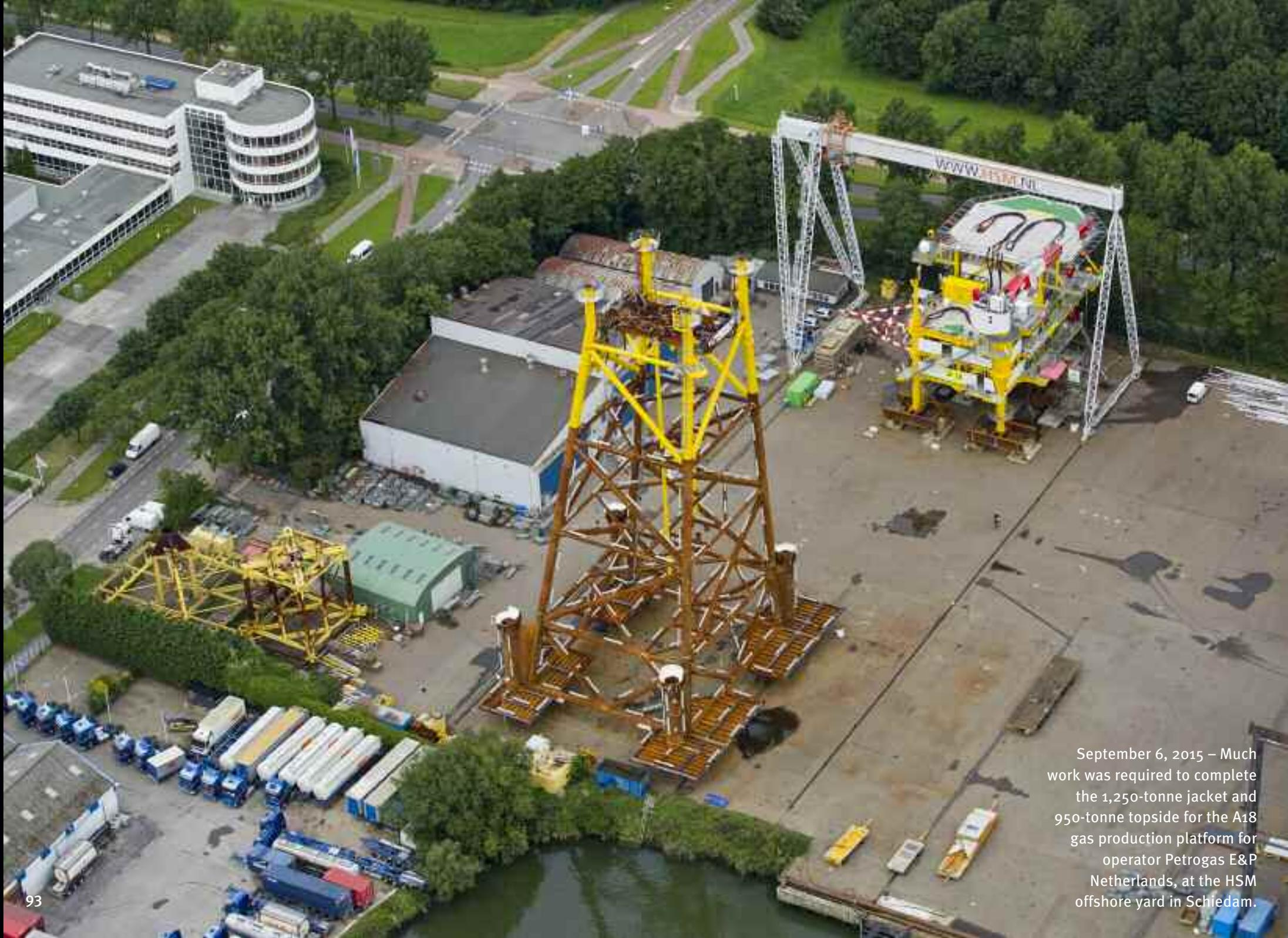
September 6, 2015 – Much work was required to complete the 1,250-tonne jacket and 950-tonne topside for the A18 gas production platform for operator Petrogas E&P Netherlands, at the HSM offshore yard in Schiedam.
