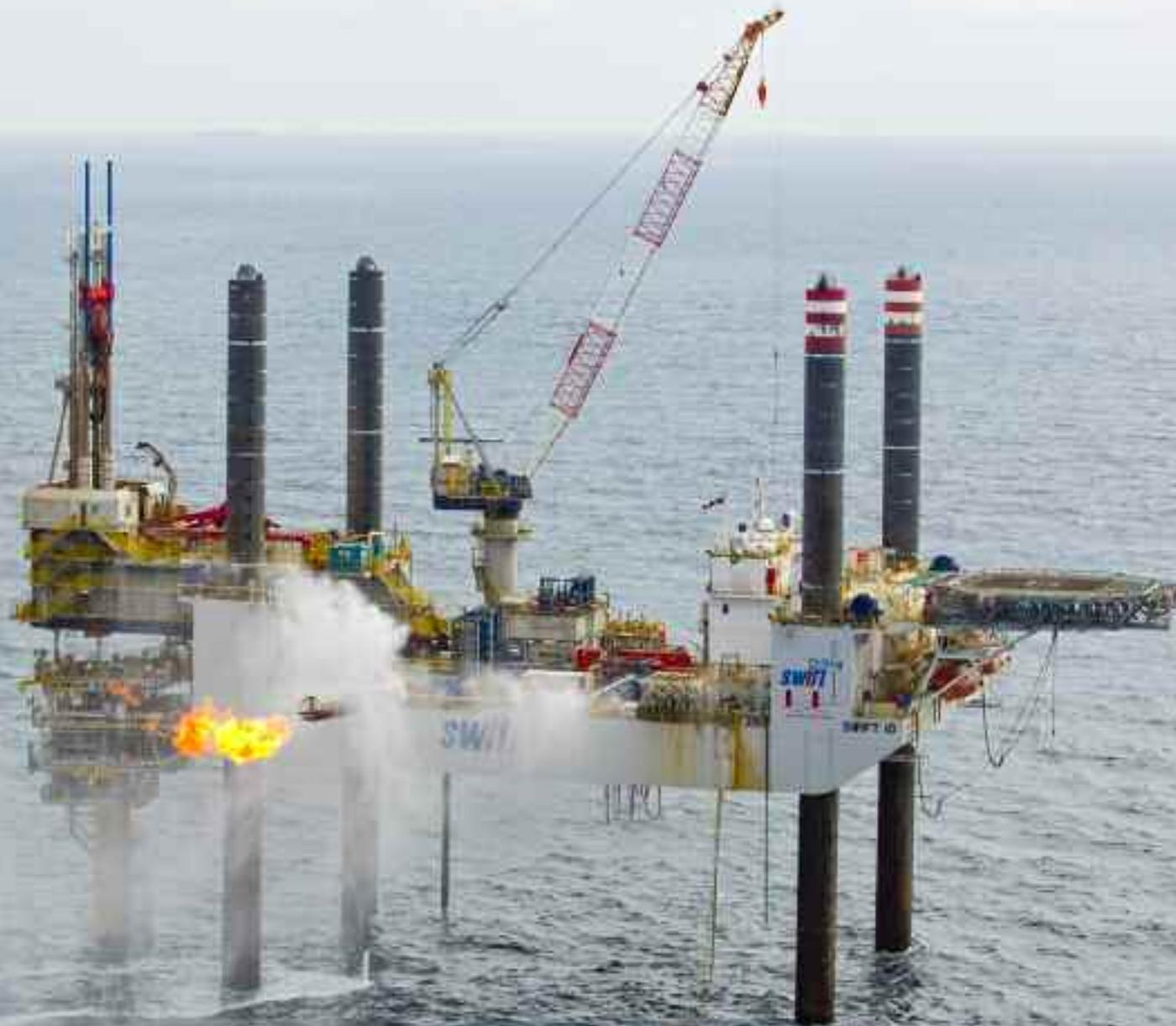
May 27, 2015 – Via the flare boom on the rig Swift 10, gas is flared as part of the testing of a gas production well at NAM's monopile L9-A mini platform, 30 miles north of the Wadden Island of Texel.
