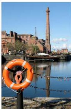
The Pump House.
