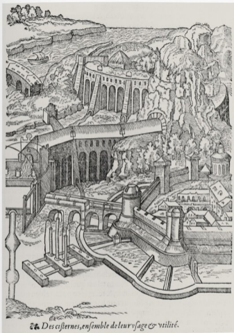
2 | Landscape view featuring dams and aqueducts To ensure a town's water supply. To illustrate Alberti's chapter "Des cisternes, ensemble de leur usage et utilité," the French edition depicts a town embedded in a hilly landscape with dams and aqueducts. In: L'Architecture et art de bien bastir du seigneur Leon Baptiste Albert, Paris, 1653, p. 214. Woodcut
