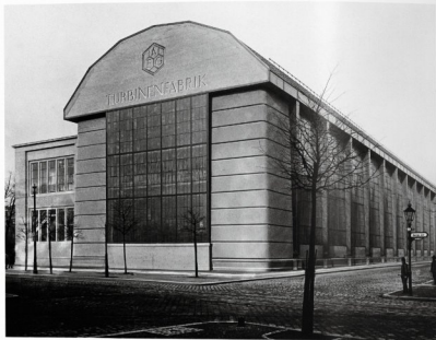
Peter Behrens (arch.), Karl Bernhard (eng.) AEG Turbine Factory Assembly Hall in Berlin, 1908-1909
